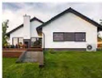
Air Source Heating
